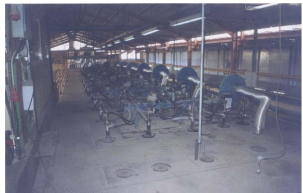
Fig. 6. Overview of the roof burners.
